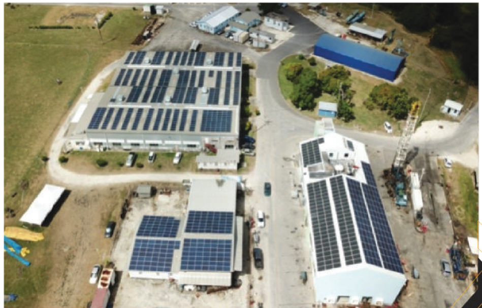
Industrial Solar Farm installation by Innogen
