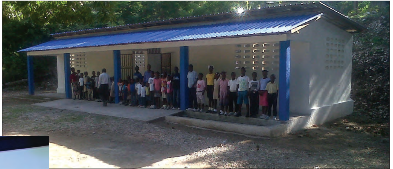
THE SCHOOL THAT WAS REBUILT AFTER THE 2010 EARTHQUAKE IN HAITI WITH FUNDS RAISED BY THE MEDIANET HAITI RELIEF FUND.
